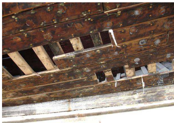
Split planks removed on starboard side
