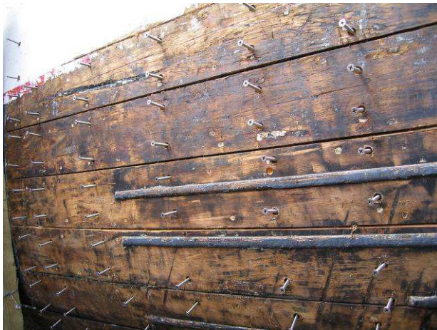
Re-screwing the planks to the rib timbers
