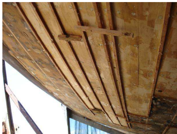
New hull planking beside the well, low down on the port side, splined and ready for sanding back.
