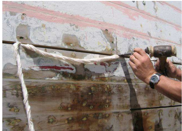
Hammering in caulking above the waterline
